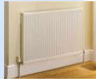
Hot Water Radiators
